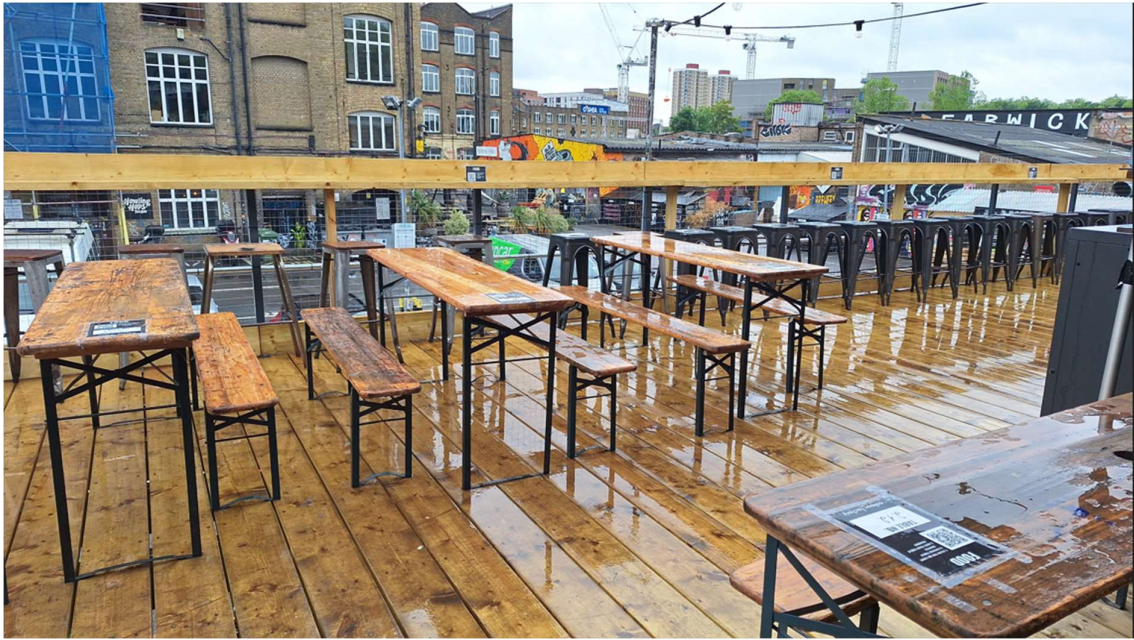
Photos – balcony area, Colour Factory, Unit 8a Queens Yard
